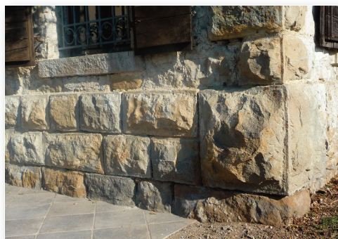
Detail of the cornerstones of the basement of the Lorenzons' house in Poffabro
