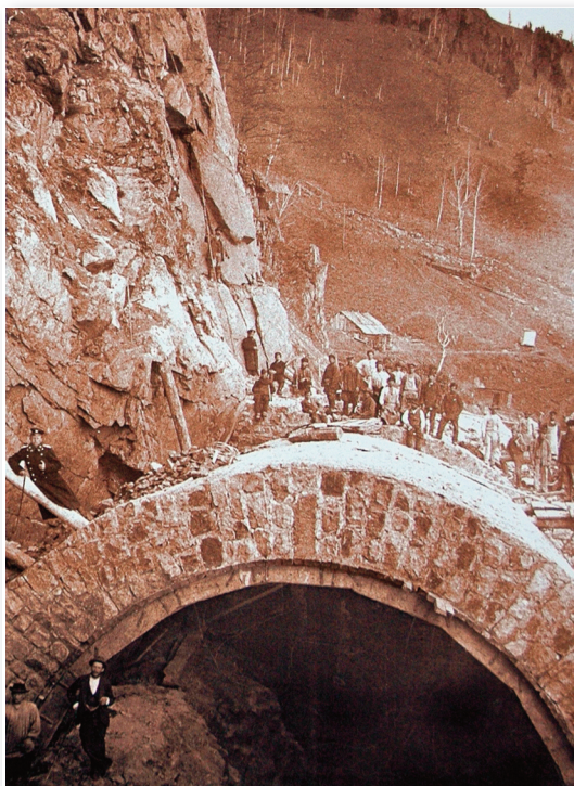
Detail of the work on the vault of a tunnel on the Trans-Siberian railway – 1904
